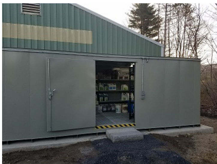
Figure 7-4. A self-contained pesticide storage unit.
