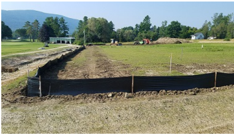
Figure 1-3. The drainage ditch was over-seeded with a erosion control mat, hay bales were placed inside the drainage ditch, and the entire project was surrounded by a silt fence prior to any construction taking place within the project.
