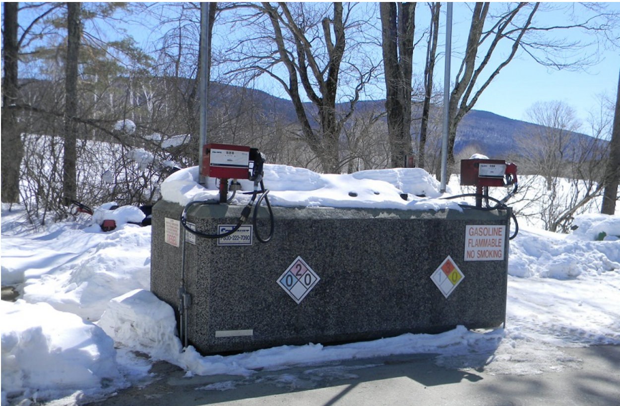
Figure 9-1. An above ground fuel tank system.
